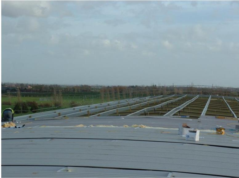
*Image 1: Undulating/out of position purlin*
