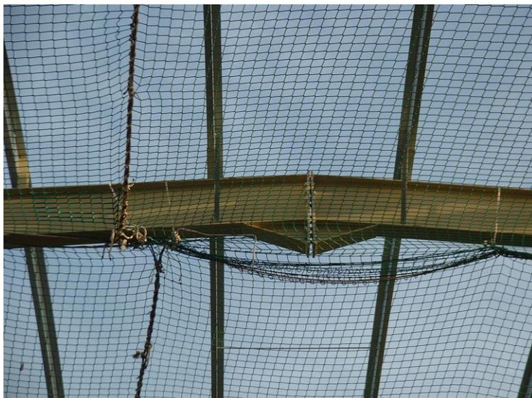
*Image 2: Incomplete structural connections*
