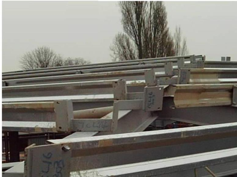
*Image 3: Incomplete structural connections*
