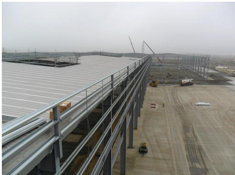
*Image 5: Primary and secondary steelwork properly installed*
