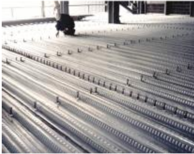
Profiled steel decking prior to concrete pour
