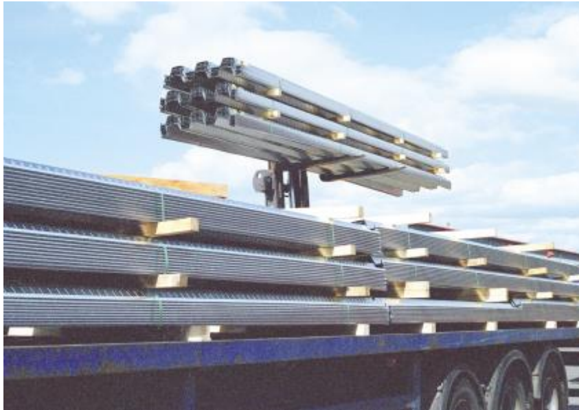
Efficient transportation of steel decking to the construction site
