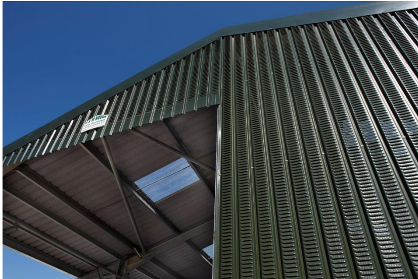
Ventair wall cladding and Dripstop fleece-lined roof panels specified for Netherton Aberdeen Angus in Perthshire. Image courtesy of Steadmans.
